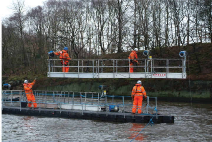
Acton Grange Viaduct
