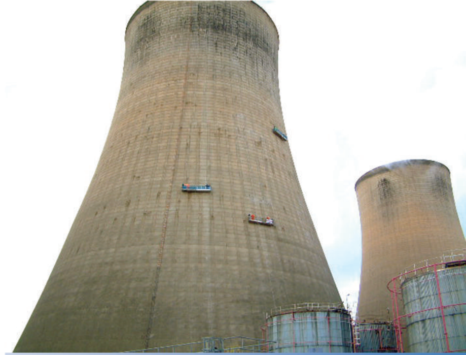
Ratcliffe Cooling Towers
