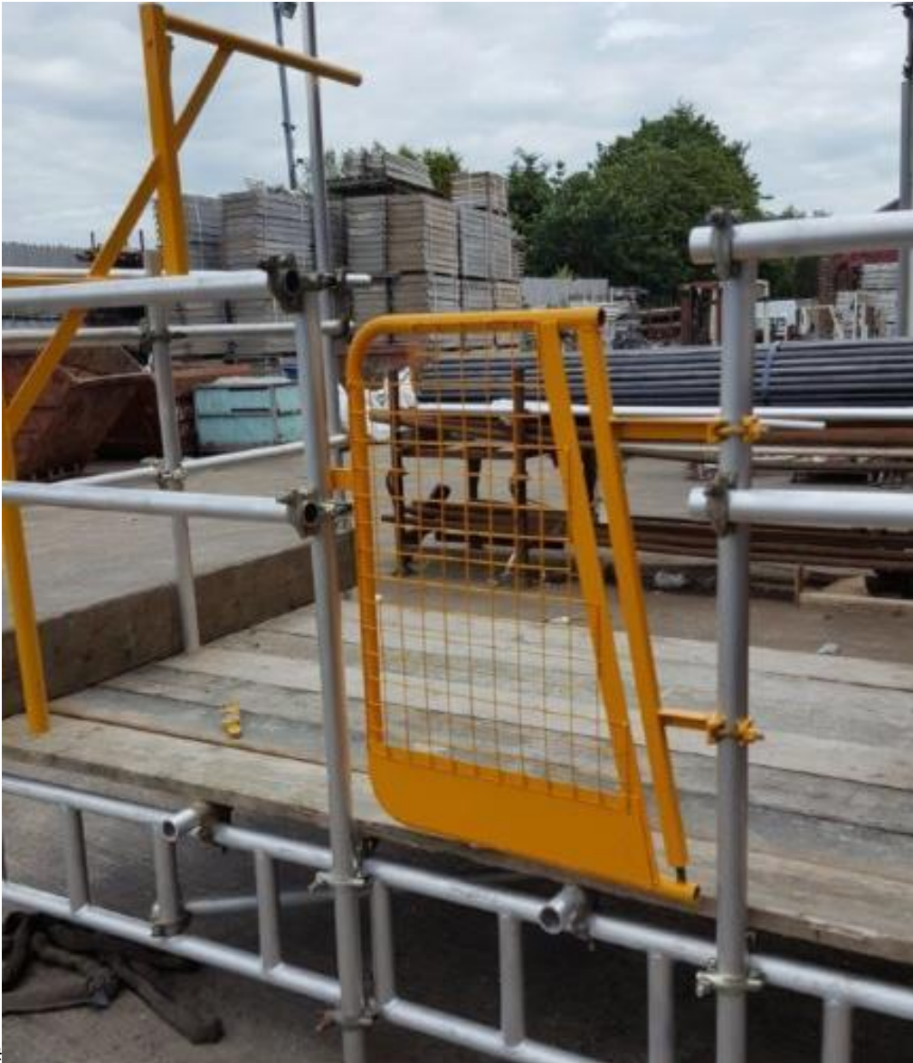
Ladder Access Gate – Drawing Number: SS0042
